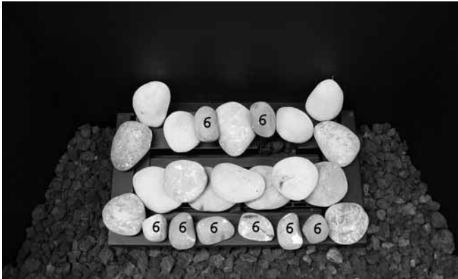
STEP 7: Place rocks #6 into position as shown.
