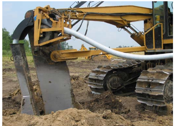
BIG O HDPE DRAINAGE TUBING IS EASILY INSTALLED
