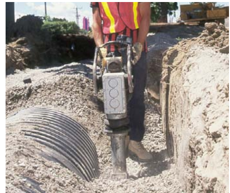
COMPACTOR PREPARING THE SOIL FOR HDPE PIPE INSTALLATION
