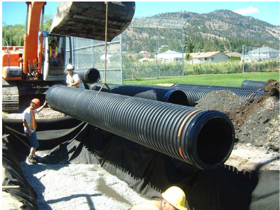
LOWERING HDPE PIPE INTO PLACE
